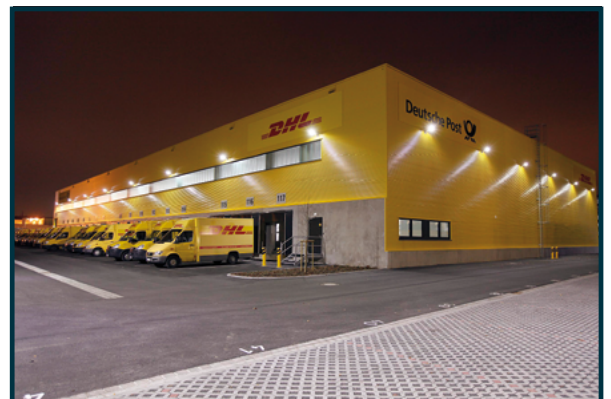
LED LIGHTING AT THE SORTING CENTRE IN HANAU, GERMANY
